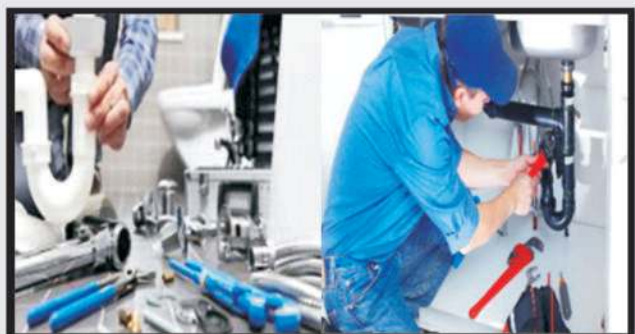
(Sanitary works Plumbers)
