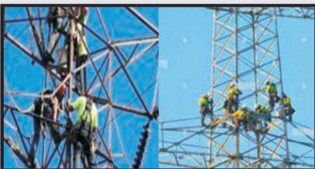
Lineman (Erectors, Cable Jointers insulators, Conductors)
